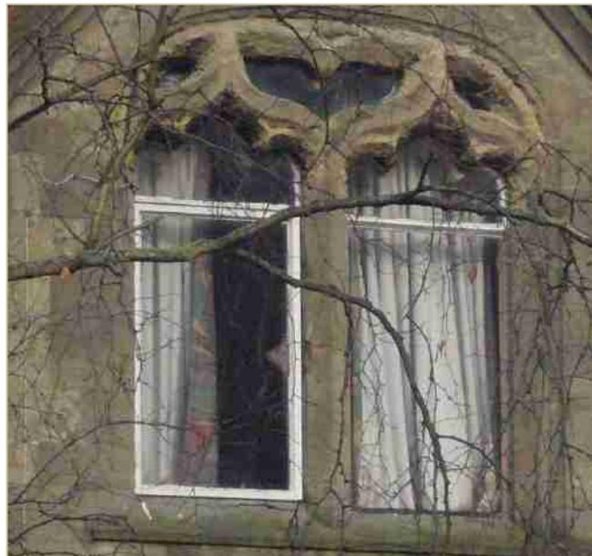
**Figure 9. Weathering to moulding on first floor of southern elevation**
