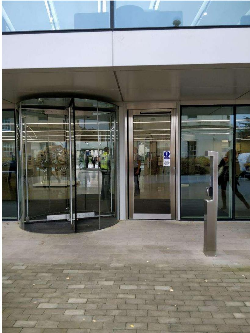
Revolving door with powered pass door immediately adjacent
