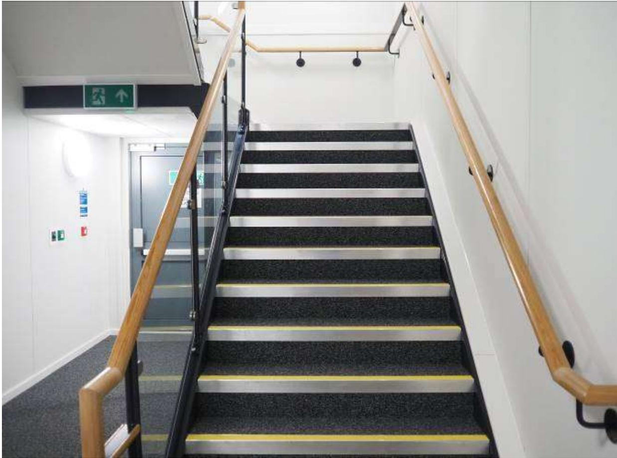
Stairs with contrasting nosings and handrails extending around the landing
