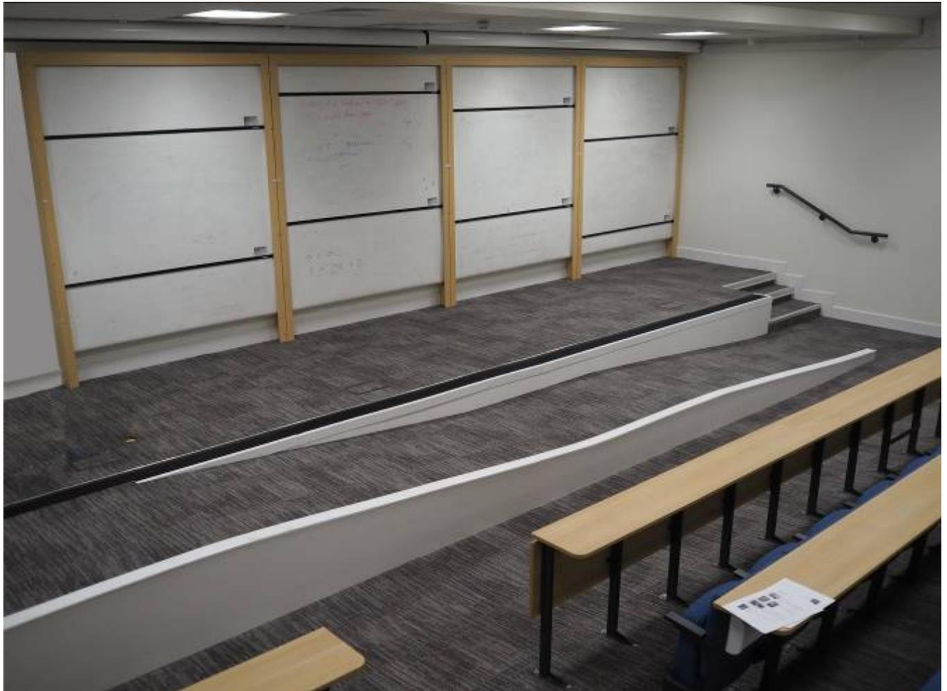
This lecture theatre has ramped access to seating, ramped access to the stage, and areas of seating that can be removed to accommodate wheelchairs
